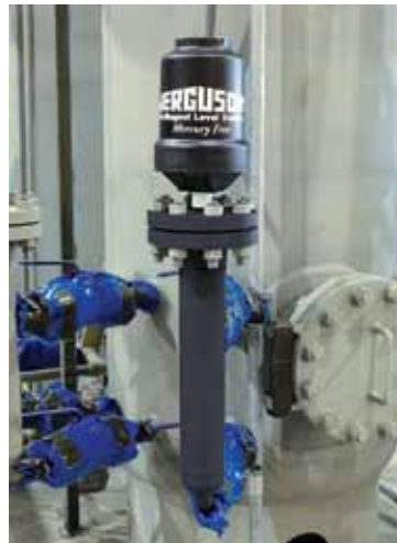
Tri-Magnet level switch and float chamber
